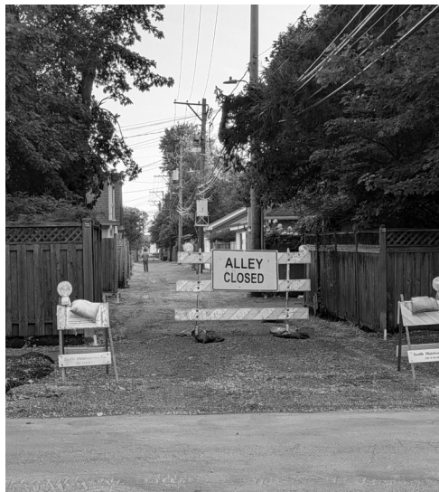
The alley during construction.
