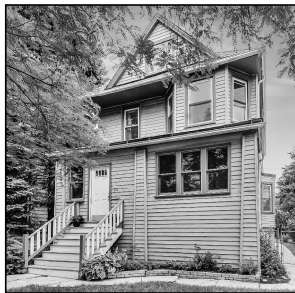
UNDER CONTRACT 4145 N Harding
