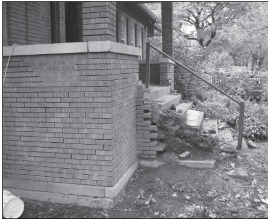
Front of Bungalow, preparation for masonry work.
